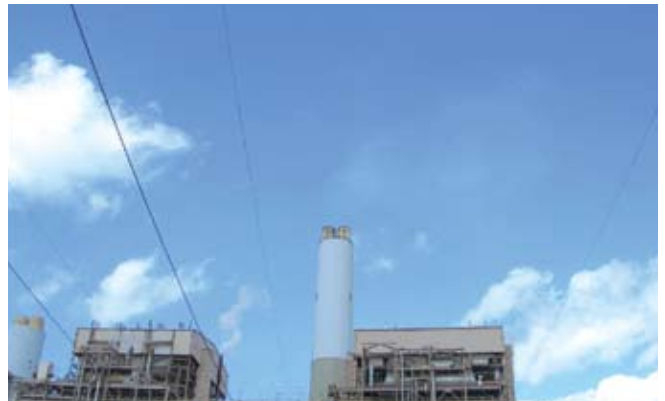
Santee Cooper, Cross Station shown during normal operations with Targeted In-Furnace Injection program on line.
